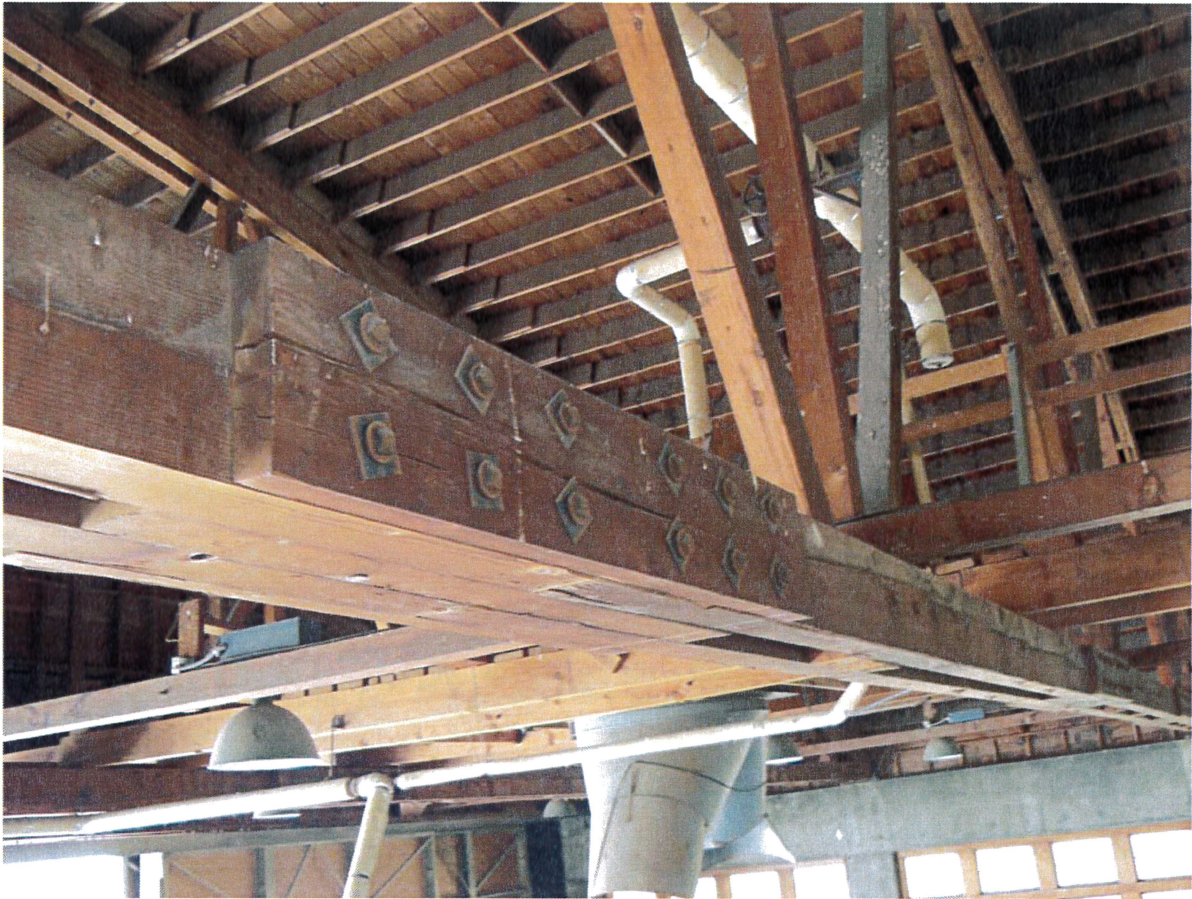
Checking in Bottom Chord (entire 20' length of board)
