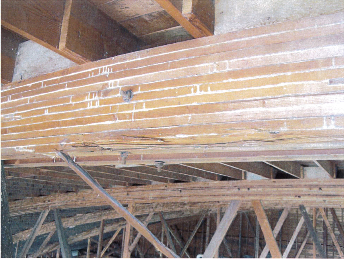
Damaged top chord
