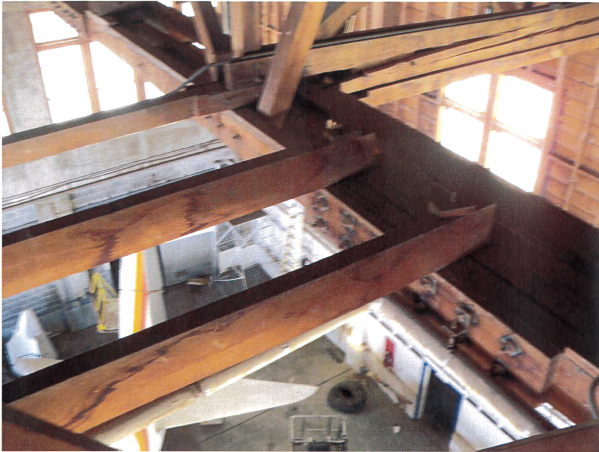
Broken Lateral Bracing
