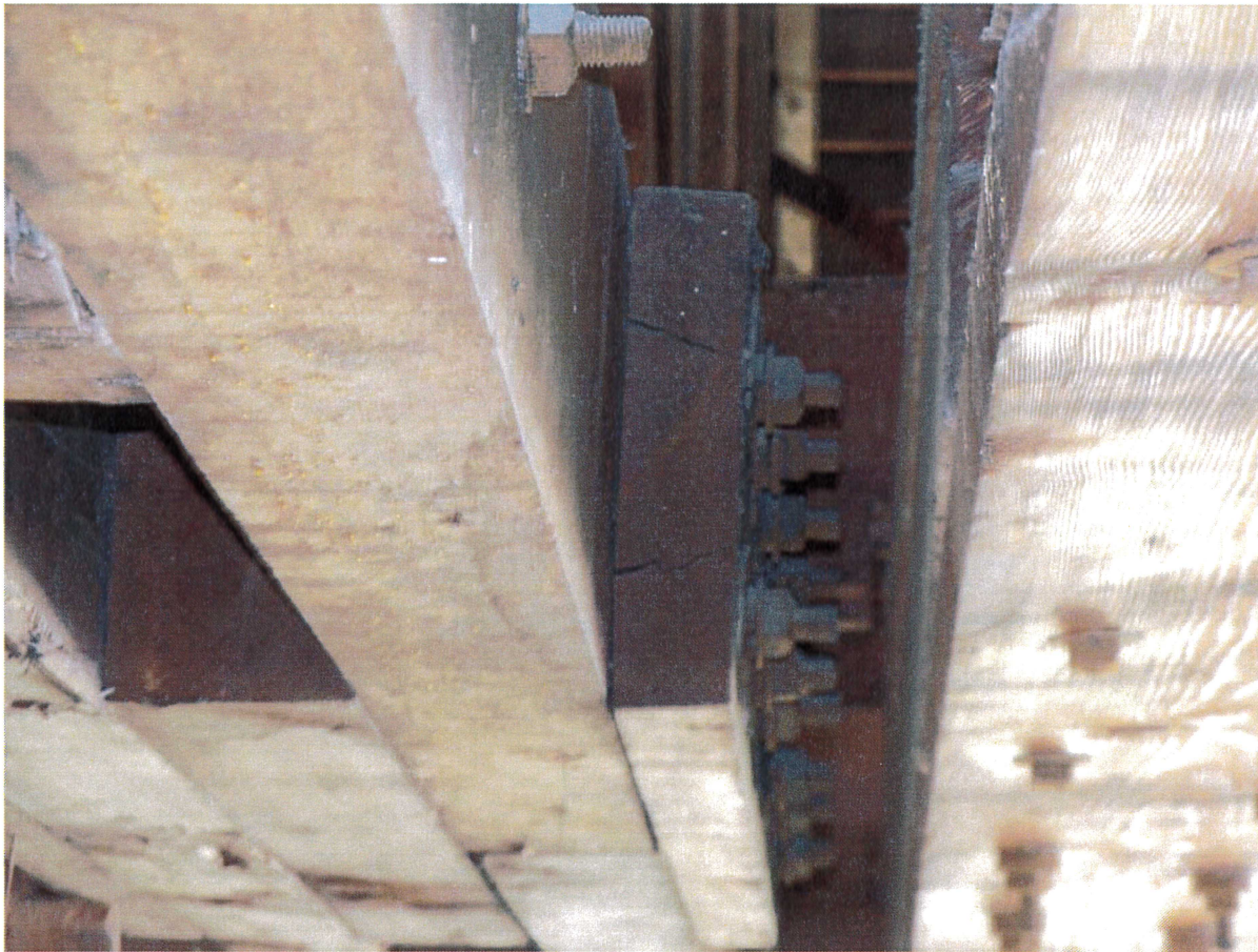
Splitting Through Splice Plates
