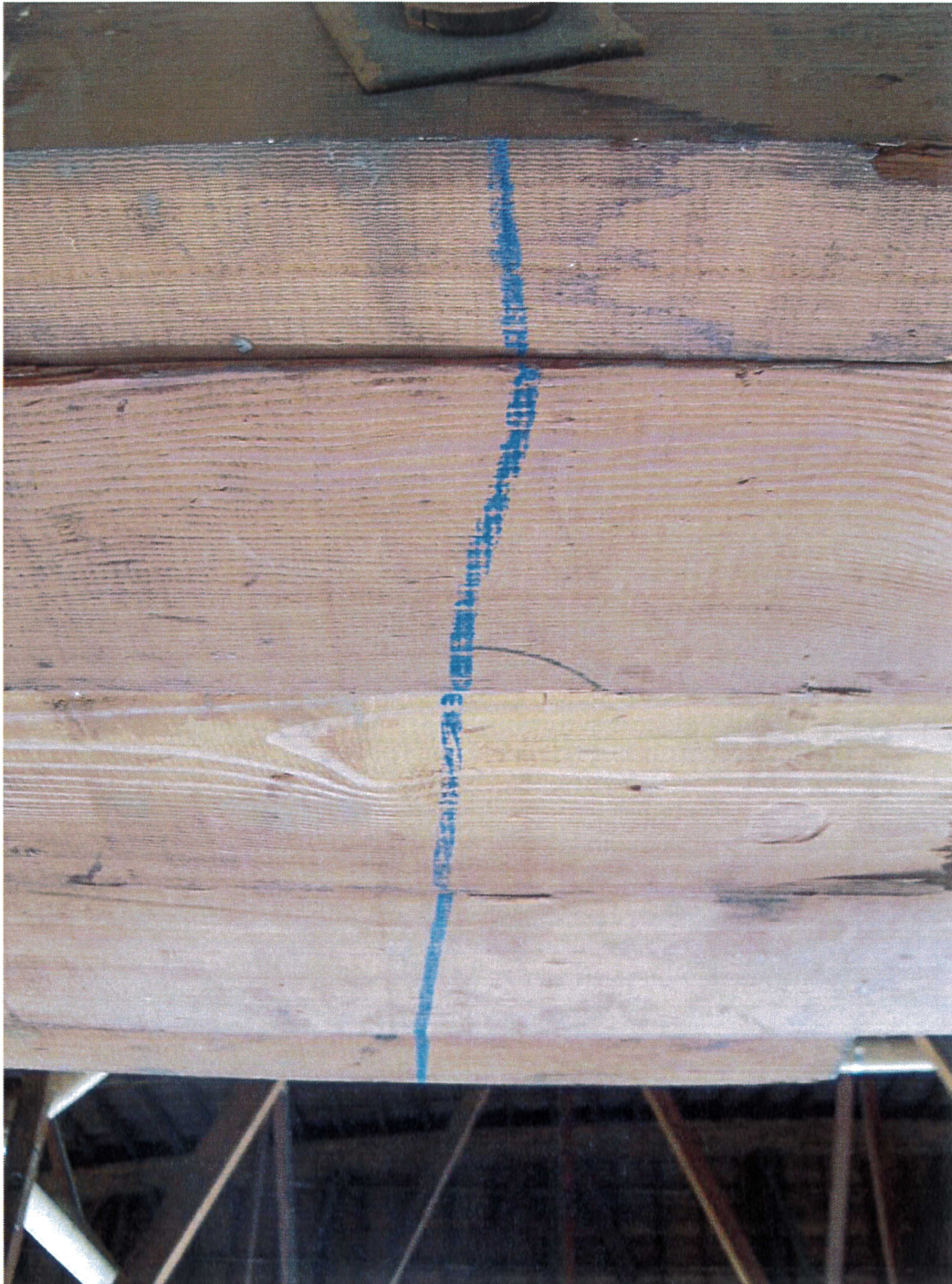
Possible Splice Plate Movement
