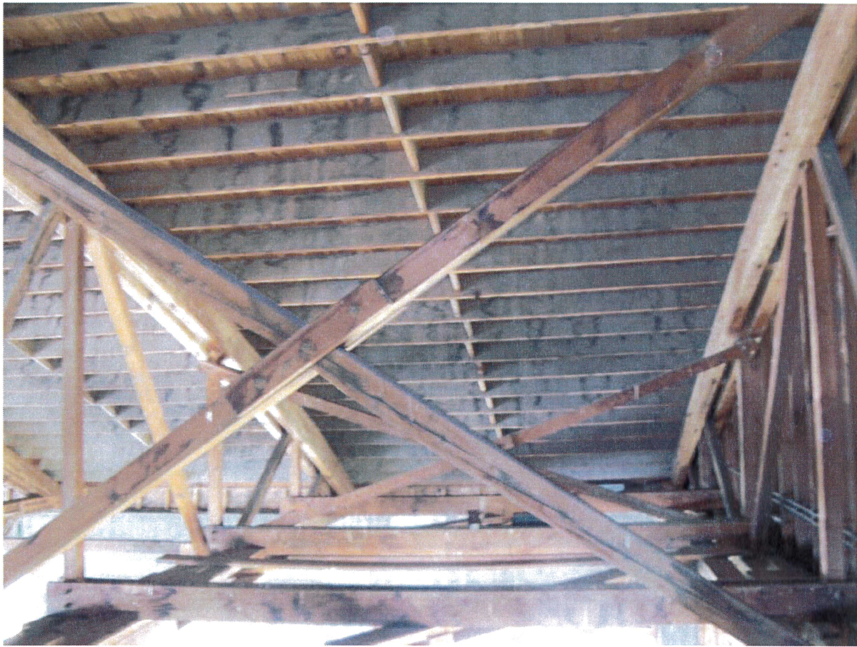
Racked and split lateral bracing
