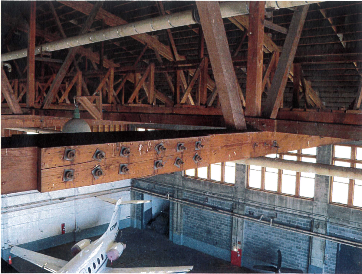
More splice plate splitting
