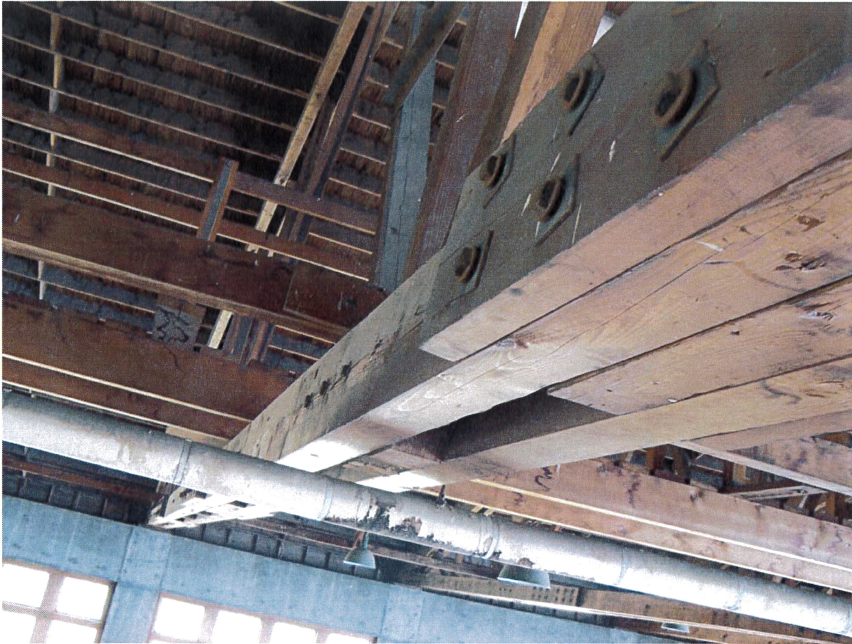
Longitudinal Splitting of Bottom Chord
