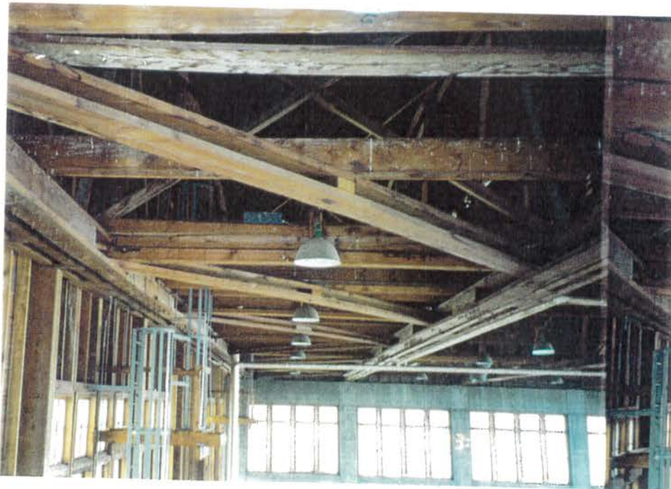
BOTTOM VIEW OF WIND TRUSS SOUTH
