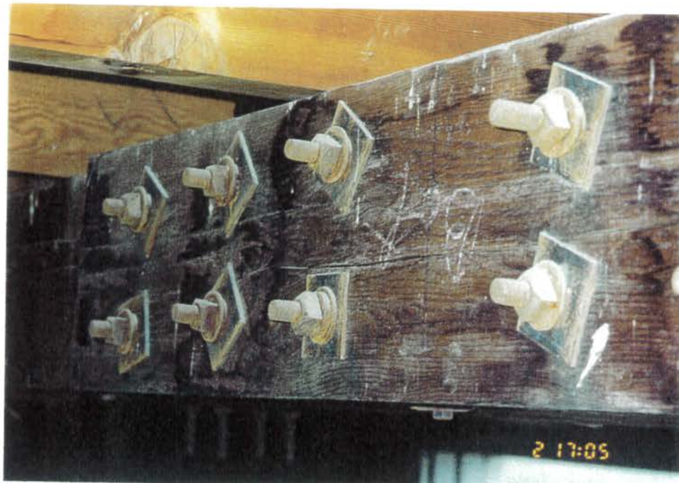
TRUSS F - SPLIT SIDE PLATE AT 5 (NOTE: SPLIT BOTTOM CHORD BEYOND)
