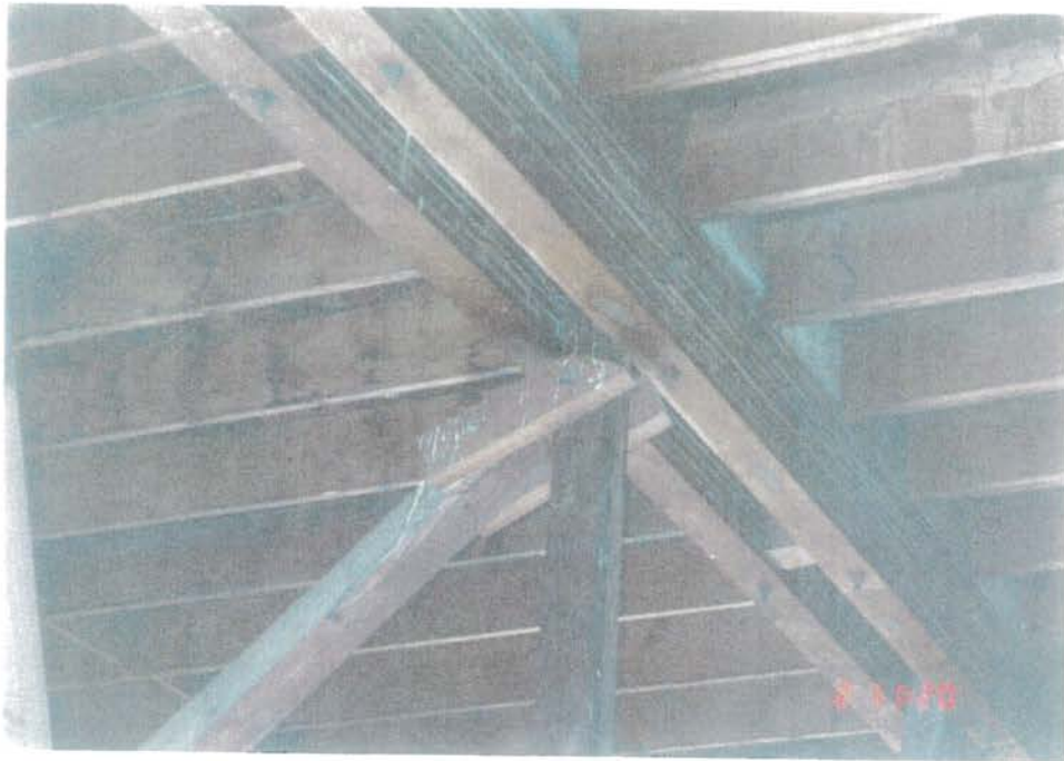
RACKED WIND "X" BRACING SOUTH
