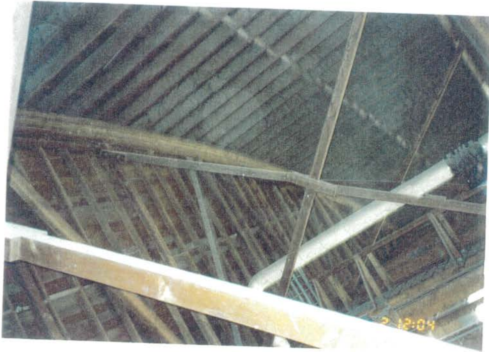
RACKED WIND "X" BRACING SOUTH
